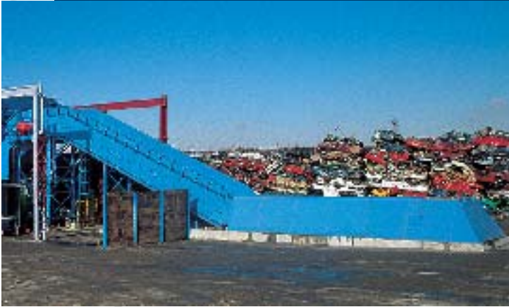
Infeed conveyor to a 5000hp shredder (UK)
